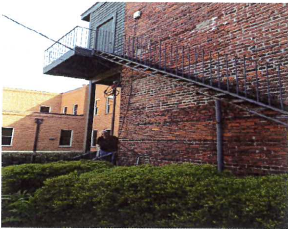
4.27 SECOND FLOOR FIRE ESCAPE
