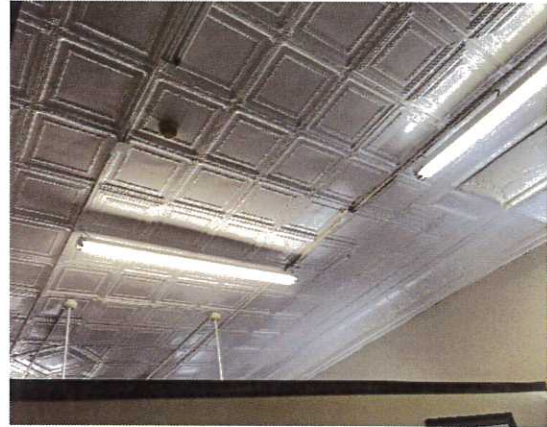
4.2 FIRST FLOOR DECORATIVE CEILING
