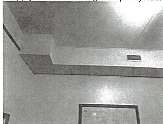
Supply duct in furring
