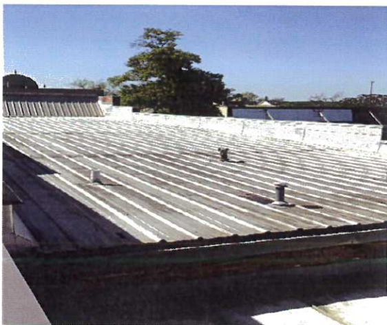
4.29 EXISTING METAL ROOF
