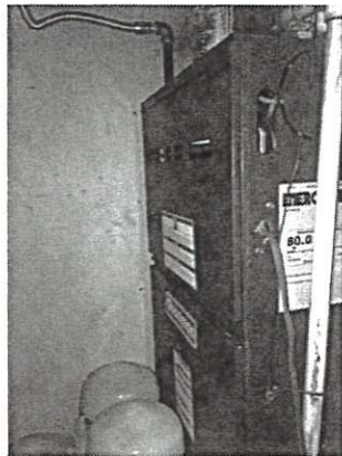
5-ton split-system gas furnace
