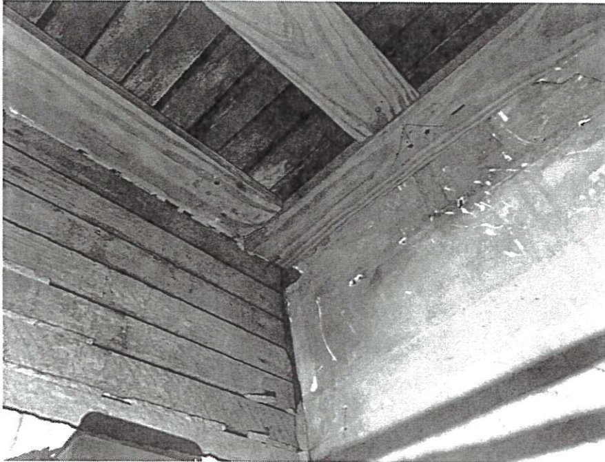
Picture No. 5 – Wood Lath and Plaster Covering Roof Framing
