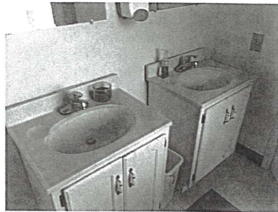
Men's room lavatories
