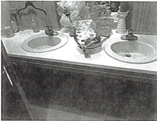
Women's room lavatories
