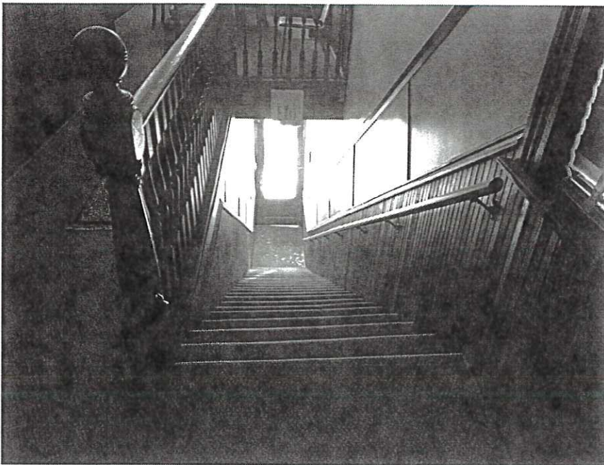
Picture No. 6 – Interior Stairs
