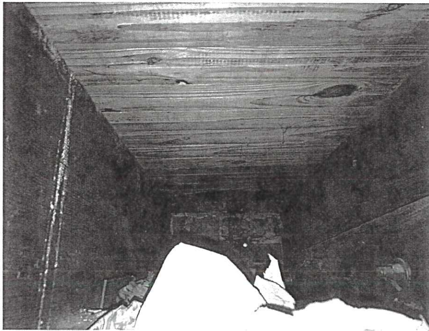
Picture No. 4 – Location of Second Floor Framing Observation
